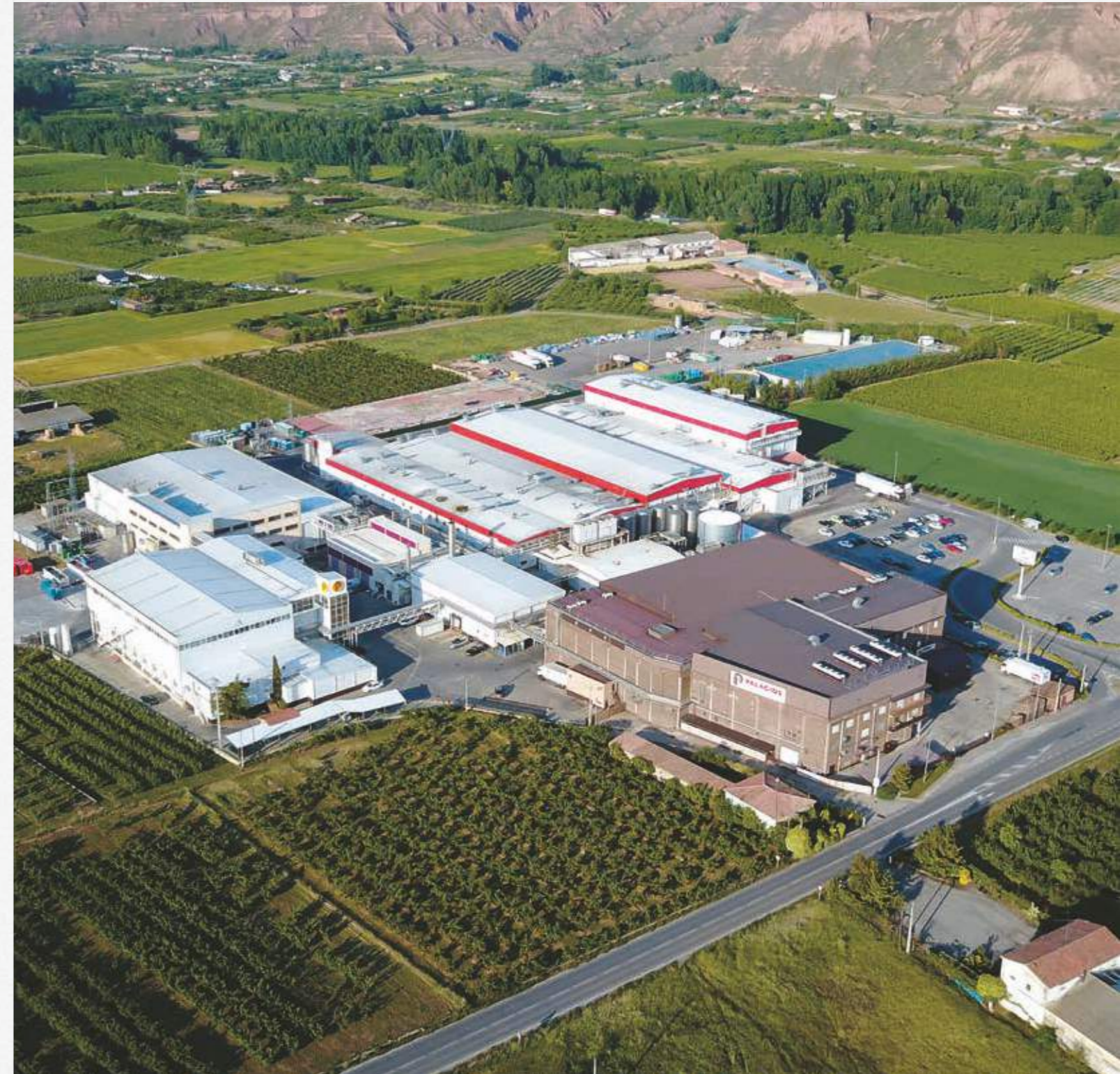
Factory in Albelda de Iregua, La Rioja, Spain.
